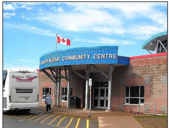
The Dr. Carson and Marion Murray Community Center houses an NHL size ice rink and saves $70,000/year in energy costs and $45,000/ year in maintenance when they switch to minewater geothermal heating and cooling. Photo courtesy of www.worldisround.com
