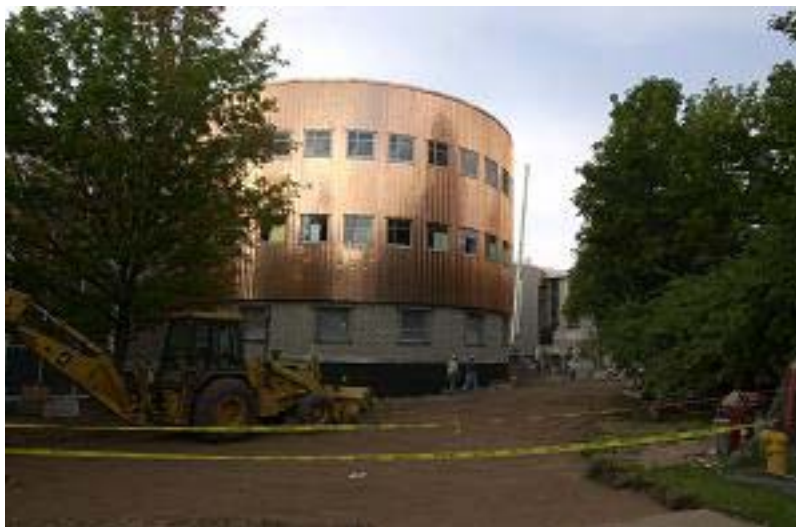
Construction of the Ann and Kanwal Rekhi Computer Science Hall
