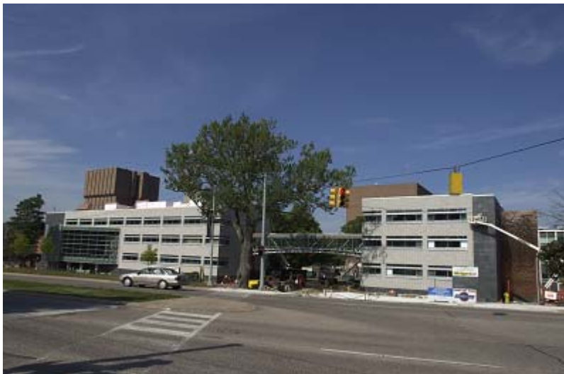
Construction of the Ann and Kanwal Rekhi Computer Science Hall and the John & Ruanne Opie Library
