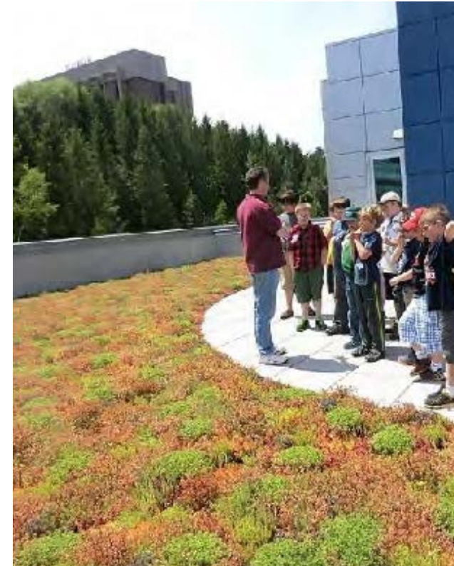
A carpet of plants on many of the second-floor roofs at the GLRC soak up runoff and act as natural temperature regulators—helping to keep the building cool in the summer months.
